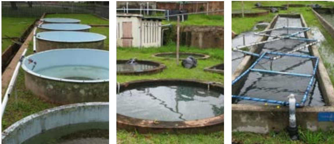
Figure 56: Outdoor round fibreglass tanks (left), outdoor round concrete tanks (middle) and outdoor raceway (right)
