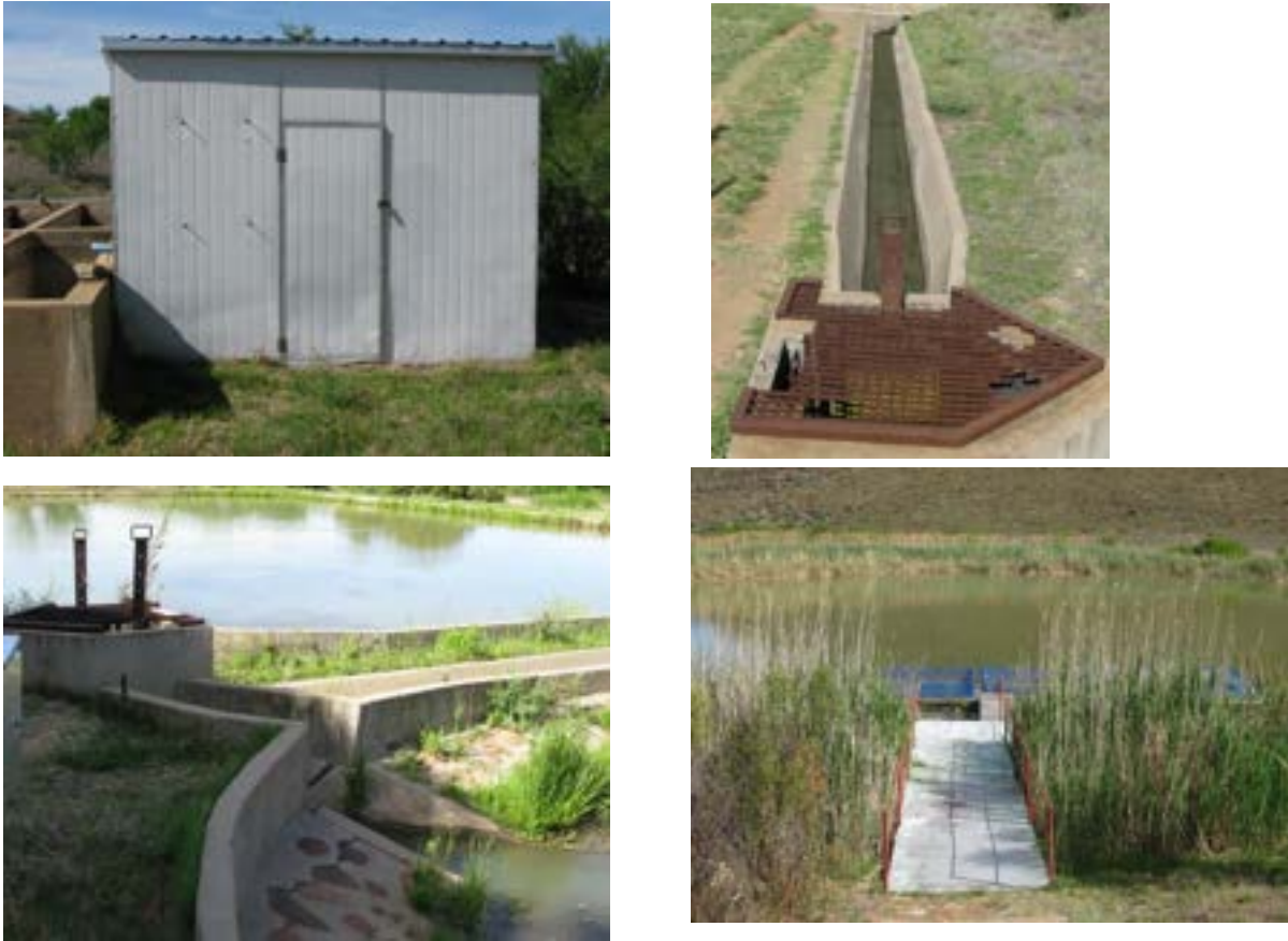
Figure 107: Incoming water filtration room (top left), main incoming water canal (top right), incoming water canal junction (bottom left) and the incoming reservoir to the fish cages (bottom right)
