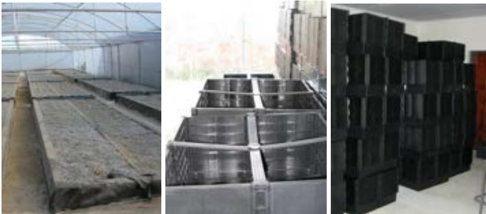
Figure 78: Aquaponics facility with grow beds (left) and grow bed containers (centre and right)
