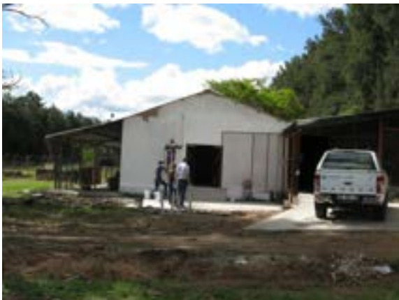
Figure 68: Construction of the new UMP Rivers of Life Water Resource and Fisheries facility
