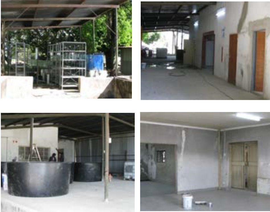
Figure 73: Facilities under construction for the new facility
