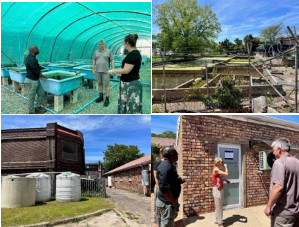
Figure 13: Various structures at DIFS, including concrete tanks, tunnel structures and laboratory buildings
