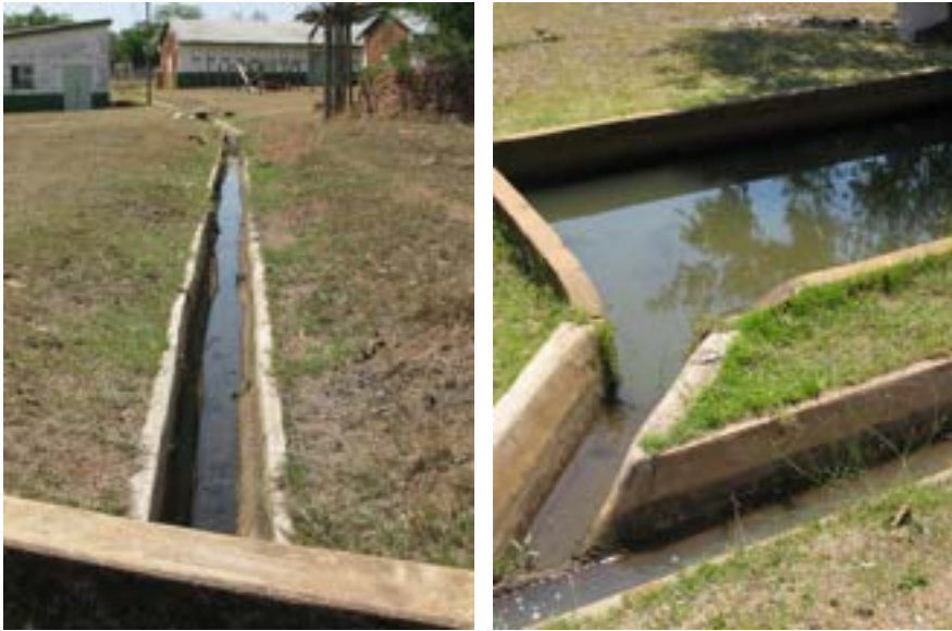
Figure 92: Open channels through which incoming water flows towards the ponds (left) and the junction between the ponds and the hatchery's water supply
