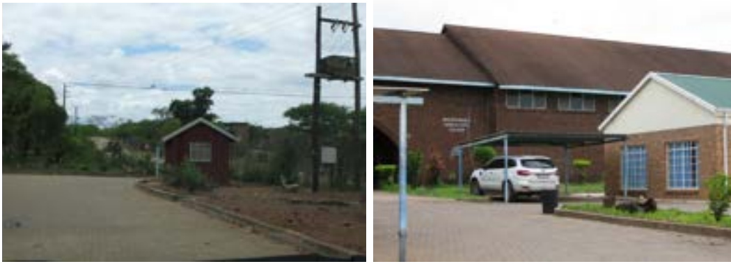
Figure 82: Security entrance (left) and main administration building (right)
