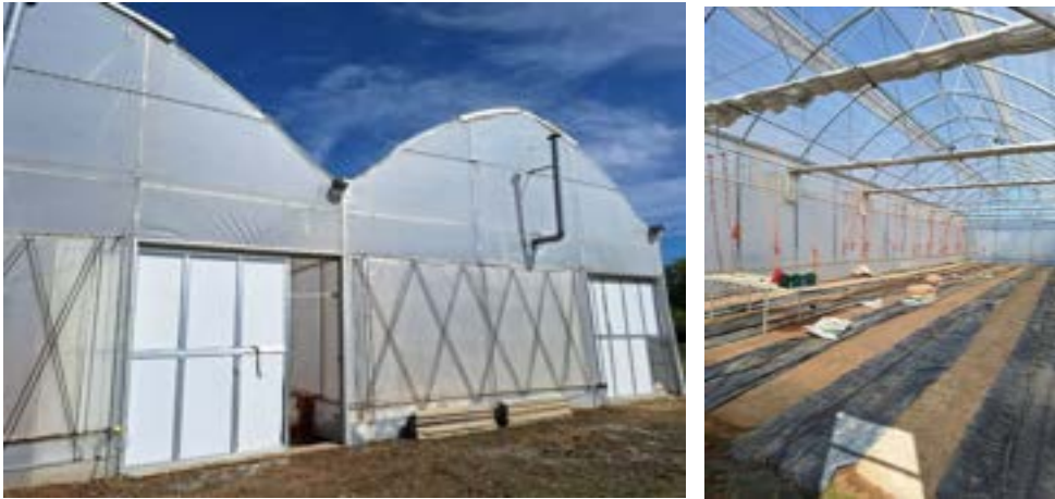
Figure 116: The tunnel structures earmarked for the Aquaculture Research Unit
