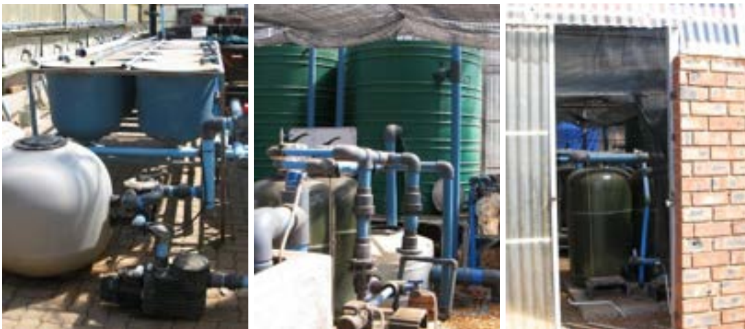
Figure 39: Water filtration systems showing sand filtration infrastructure
