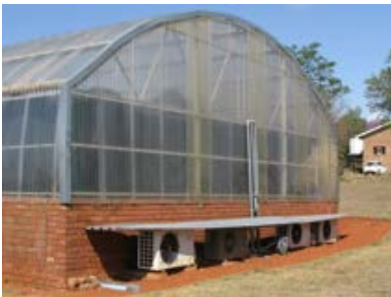
Figure 43: Heat pump systems installed on the new tunnel (left) and the new tank systems installed for the new tunnel (right)
