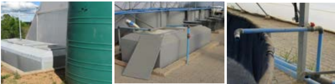
Figure 76: DARDLEA infrastructure processing facility
