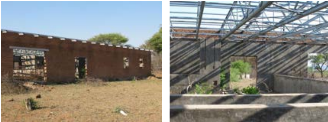
Figure 99: Partially completed fish-processing facility
