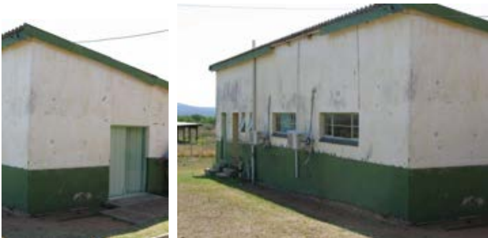
Figure 98: Aquaculture operations office building
